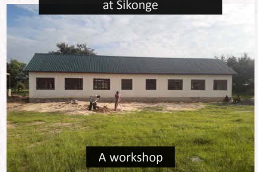
New building and rehabilitation at Sikonge
