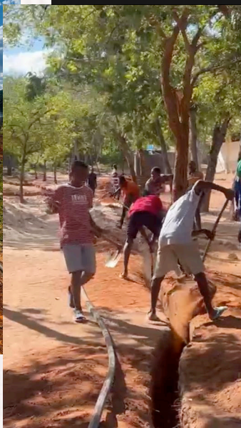
Secondary School students digging the trench for the pipe
