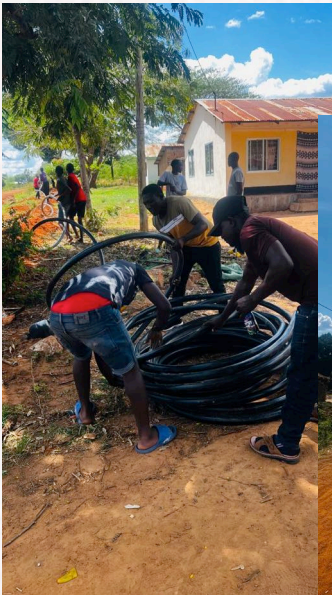
Unrolling the pipe which will carry water to Kiloleni secondary school
